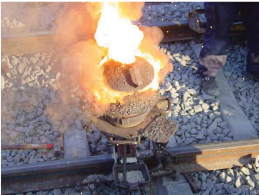
*A small clay pot contains a thermite mixture. It is reacting at high temperature in the photo and will eventually produce molten metal to join the railroad tracks below it.*
